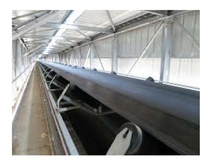
"Completely covered belt conveyors have been considered for material conveying from ship to respective storages"
