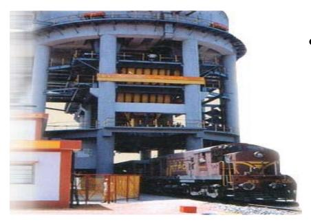
In rapid loading of material, material is loaded on rake, while the railway rake is in motion. Below the main hopper, another small hopper is provided on load cells, which can accommodate about 1 wagon load of material.
